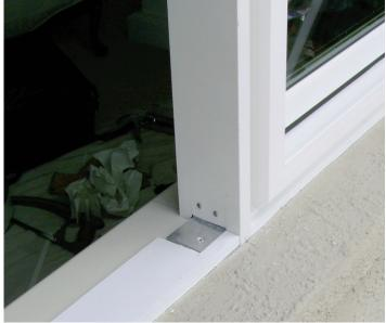
A Structural Mull is usually a piece of steel with legs at top and bottom that allow the mull to be securely fastened to the header and sill - or even to the jambs where a horizontal mull is required.
