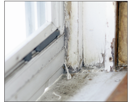
Opening and Closing Constantly Grinds Lead Dust
