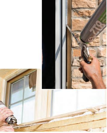
density of 1.8-2.3 pound per cubic foot (pcf), and can provide structural enhancement in certain framed buildings. The smaller cells trap insulating gas from the curing, which has a lower thermal conductivity than still air, and increases the R-value to anywhere from R5.8 to R6.9 per inch.
