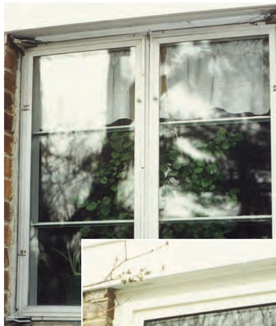
Old Steel Window in Brick Opening
