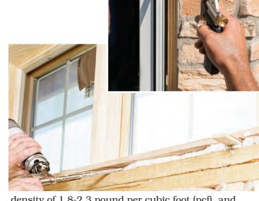
density of 1.8-2.3 pound per cubic foot (pcf), and can provide structural enhancement in certain framed buildings. The smaller cells trap insulating gas from the curing, which has a lower thermal conductivity than still air, and increases the R-value to anywhere from R5.8 to R6.9 per inch.
