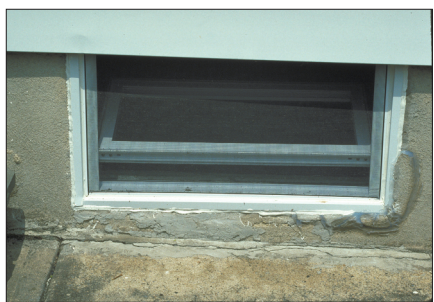
After: New Hopper Basement Window
