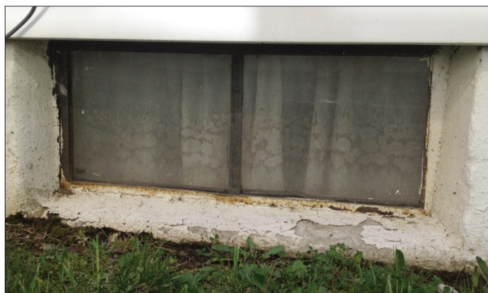
Old Steel Basement Window
