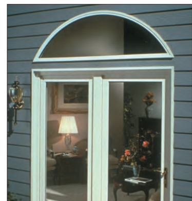
Safety Glass is Required Near Doors, Walkways and Stairways
