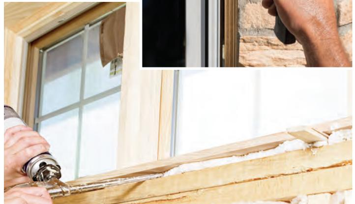
density of 1.8-2.3 pound per cubic foot (pcf), and can provide structural enhancement in certain framed buildings. The smaller cells trap insulating gas from the curing, which has a lower thermal conductivity than still air, and increases the R-value to anywhere from R5.8 to R6.9 per inch.
