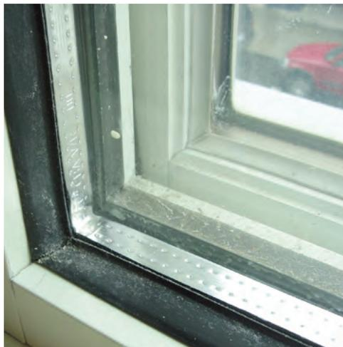
Asymmetrical Glazing (panes of glass of different thickness in one unit) is another approach to reduce sound transmission often at a lower cost than laminated glass or storm panels,
